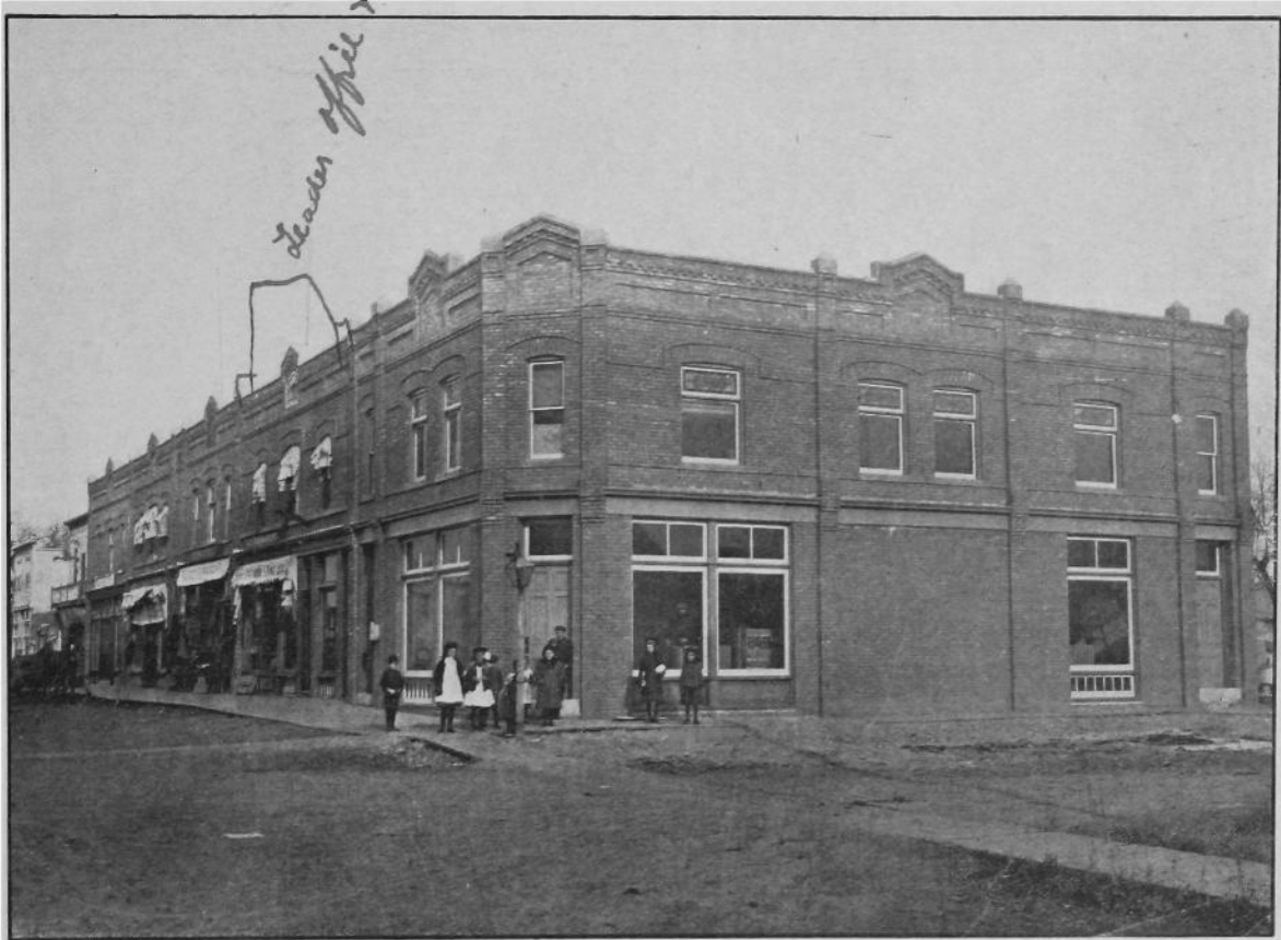
The Post Office, Leader Block and Noble Block, Villard avenue. The Post Office is the first in the row.
