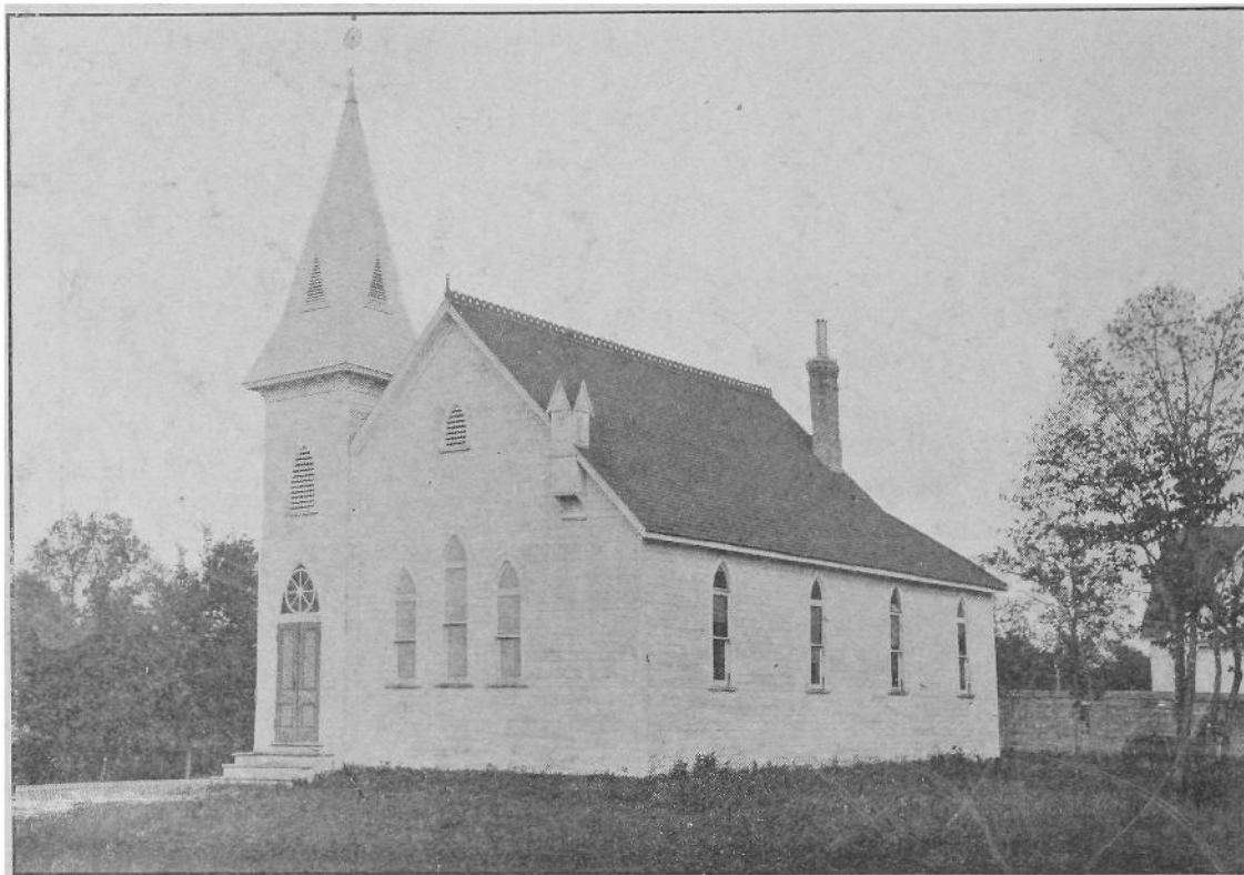
Baptist Church, corner of Browning avenue and Ash street.
