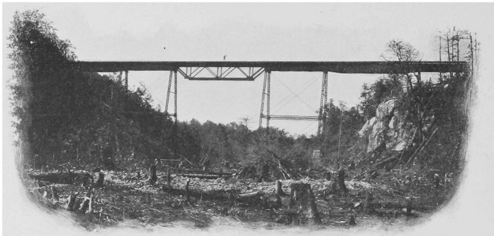
St. Flore Bridge
