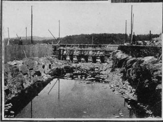
"This canal is 1000 feet long by 100 feet wide and 20 feet deep, and was excavated out of solid rock"
